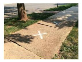
The inspector marks an orange [X] or  $[X > \langle X]$  for a continuous string of defective sidewalk squares which meet one or more of the following criteria:
